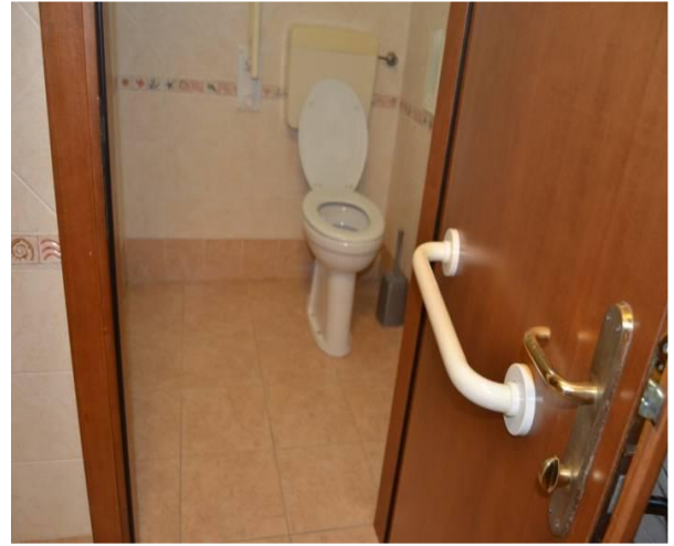
59 Toilet with grab bar
