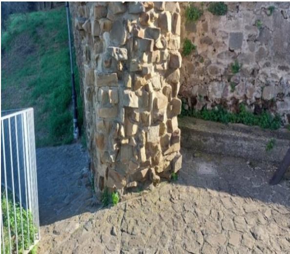
42 entrance passage from the ramp to the terrace
