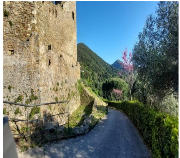
49 last section of the asphalt ramp
